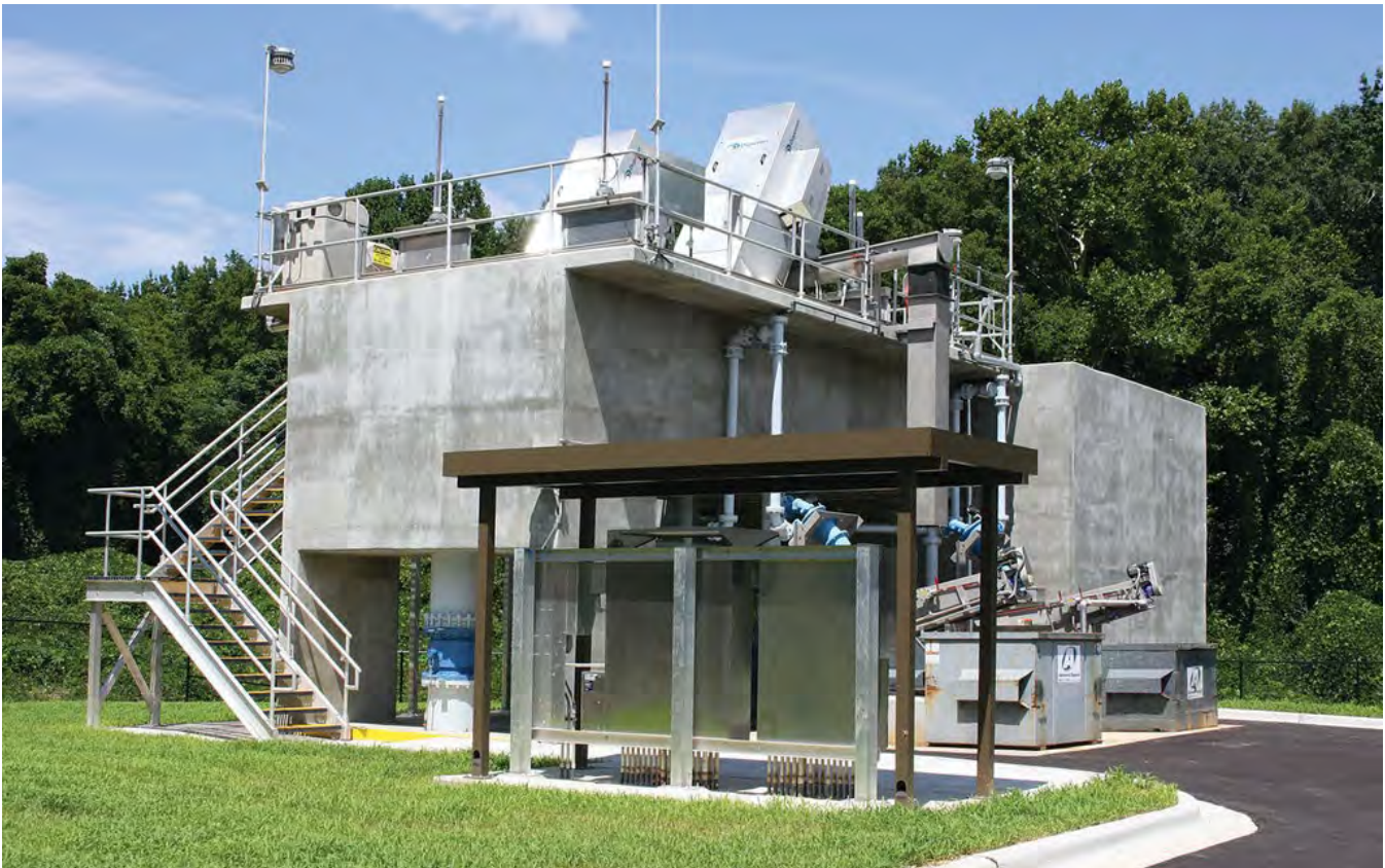
New headworks added as part of the Pine Creek Wastewater Treatment Plant upgrades
